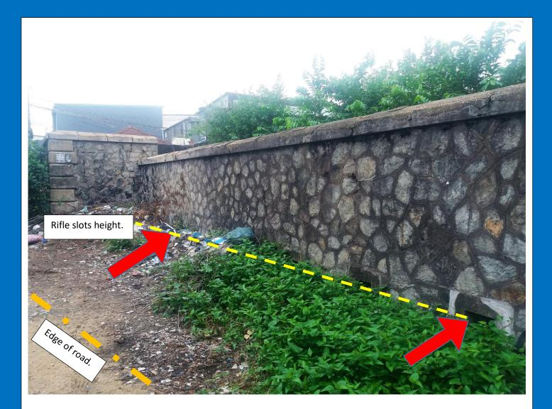
Part of the exterior of the northern wall. It runs parallel to the small road. Over time, the road height was raised about four feet. Therefore the blockhouse was actually four feet higher than it appears. The rifle slots should be about four feet above ground level.
