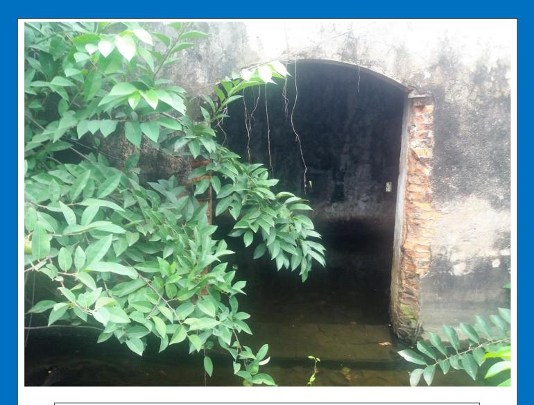
When entering through the gate there is about 10 metres to this wall straight ahead. The wall holds up a mezzanine floor, which runs around the inside of the blockhouse. Arches along this wall give access to a series of separate rooms with rifle slots (accommodation?).
