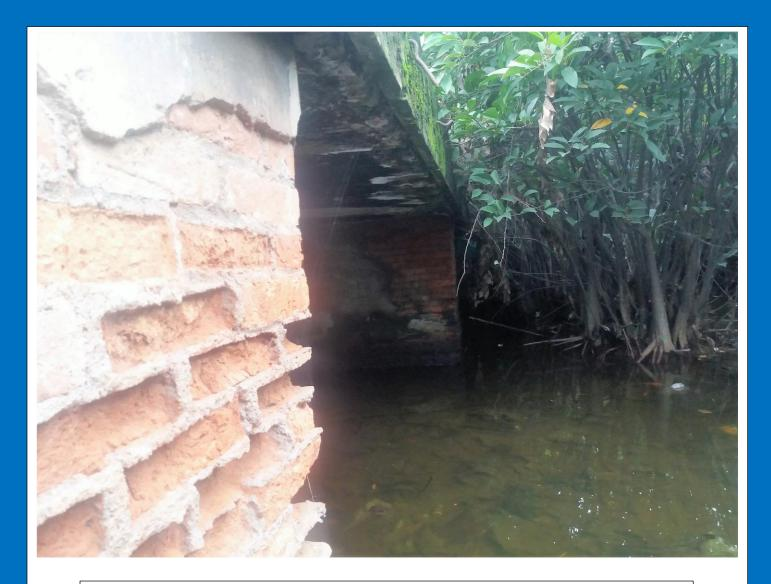
As I entered through the gate; to the left is one of the pillars supporting the mezzanine floor attached to the northern wall. The pillars are of clay bricks. When the French arrived they found six clay fields, and two more clayfields suitable for furnace-bricks. Therefore high quality clay bricks and tiles are a feature of French military and civilian architecture. Here is a close up example.
